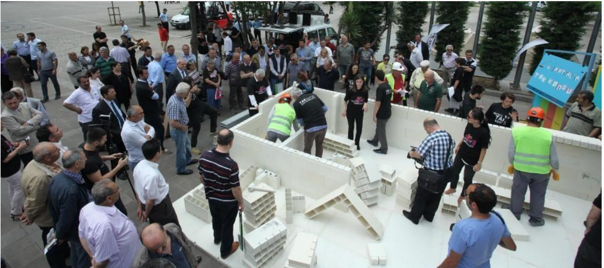
TAK Kartal Sales Office (Finished in 7 days)
