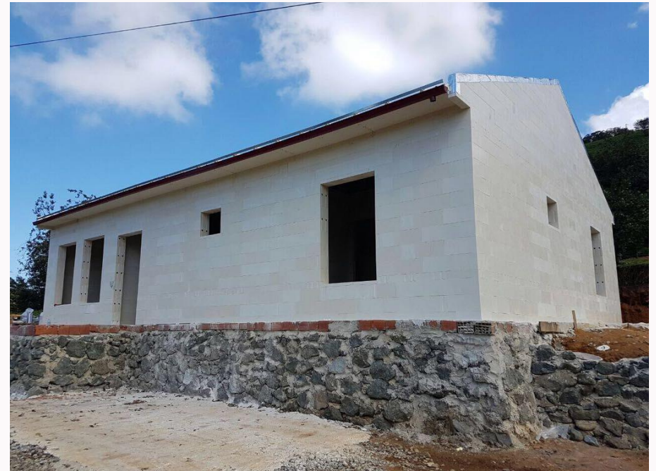
Shell Construction of a 1100 sq feet House (Finished in 3 days)
