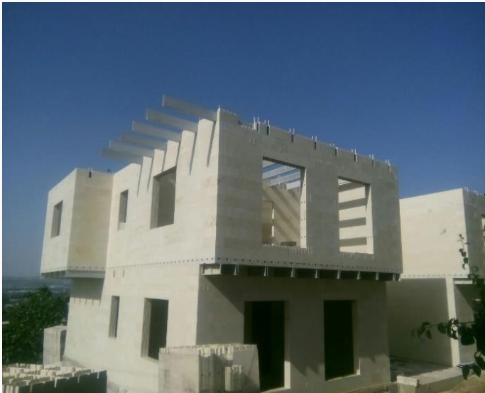
Shell Construction of a 4400 sq feet House (Finished in 7 days)
